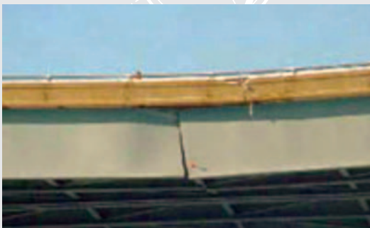
Small, previously monitored brittle cracks in the Hoan Bridge support span girder webs rapidly propagated on a cold December morning during a period of heavy vehicle traffic.
