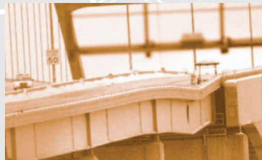
Small, previously monitored brittle cracks in the Hoan Bridge support span girder webs rapidly propagated on a cold December morning during a period of heavy vehicle traffic.
