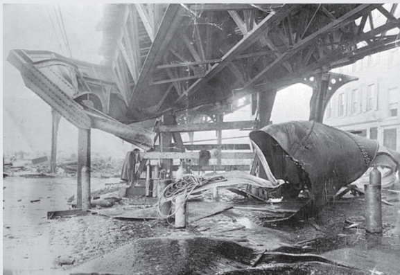
Destruction of the elevated train overpass after impact by sections of the storage tank and the tidal wave of molasses that followed. Although not confirmed, the twisted piece of riveted metal plates at the right may be part of the tank.
